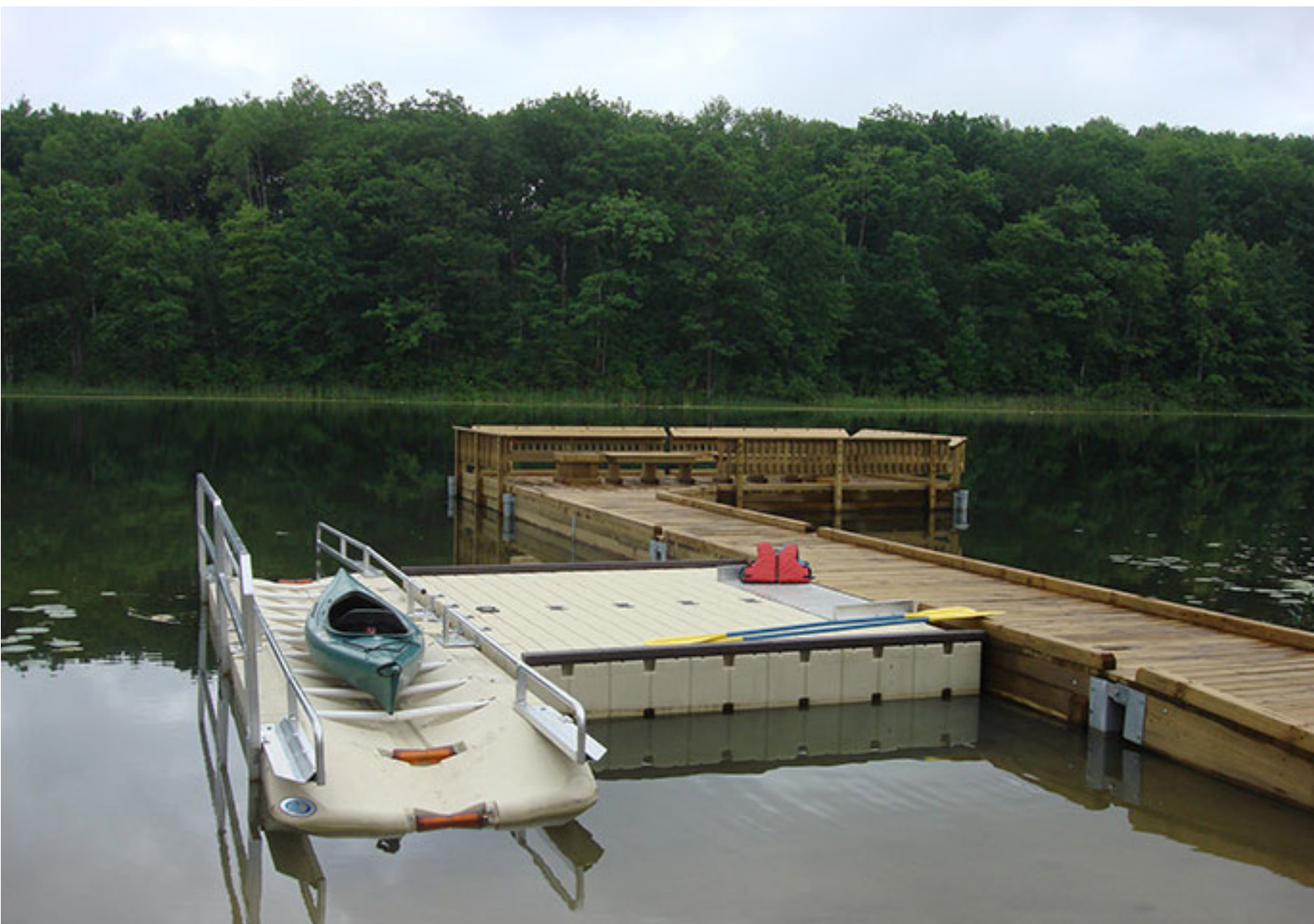
Figure 40. The new launch ramp at Grebe Lake in the Rifle River State Recreation Area Credit: Michigan Department of Natural Resources
