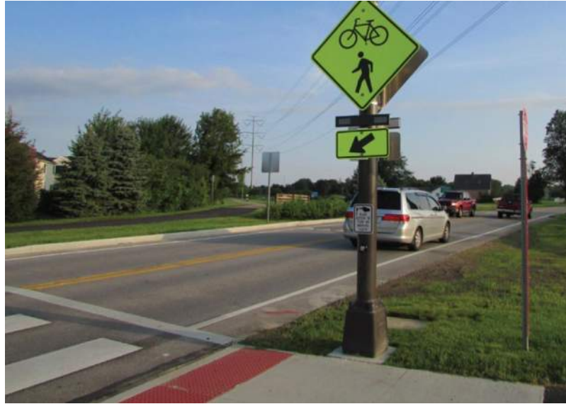
RECTANGULAR RAPID FLASHING BEACONS (RRFBs)
