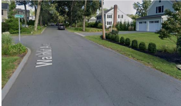
Walnut Avenue near Cheever Circle, looking east
