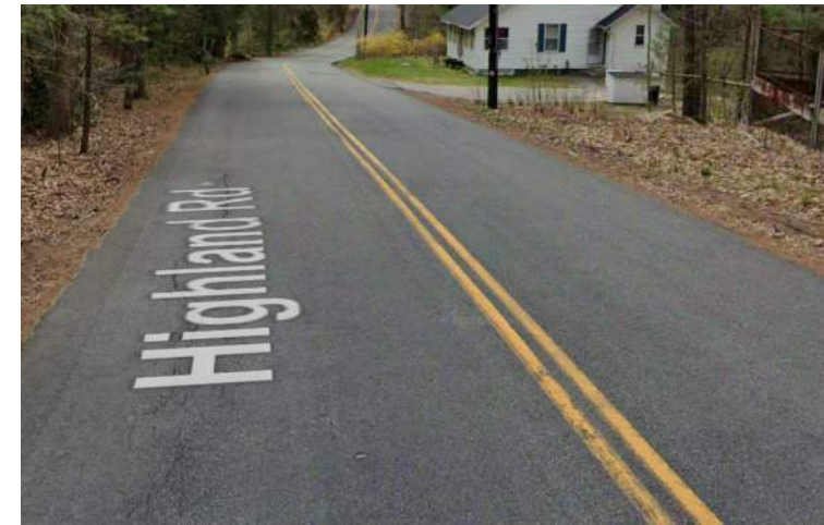
Highland Road near Woodland Road, looking south
